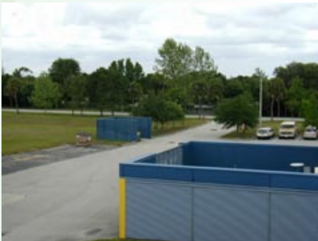
Figure 7. The blue enclosure in the background allows trash dumpsters to be kept away from the facility.
