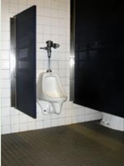
Figure 23. Stalls and partitions should be suspended from the ceiling or extend from a wall to permit easy floor mopping and reduce build-up of soil on legs and other floor supports.
