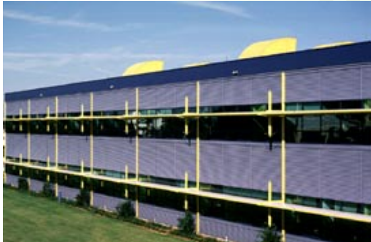
Figure 19. Window shading devices can be incorporated into the architecture of a building, such as these exterior light shelves at the Florida Solar Energy Center in Cocoa.
